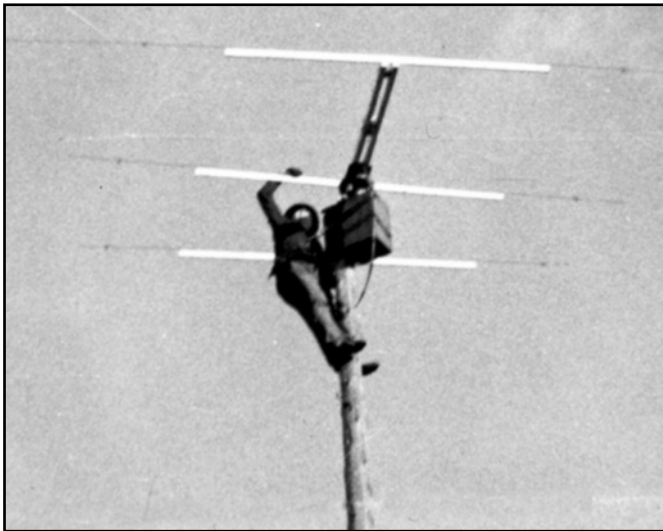
Jim MacGregor, W8DUA, in this c1947-dated photo is shown servicing a classic "33" beam and homebrew rotator atop a 50-ft, utility-like pole in his home's backyard on Fletcher Ave., Kalamazoo. Jim made use of a washing machine motor in the approximately 40-lbs. homebrew rotator, encasing it in metal. Installing the rotator atop the pole - and then further mounting the beam antenna above it - was a nightmarish challenge.
