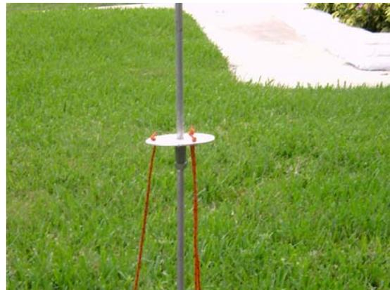
The picture on the left is the die that Tom used to cut the threads into the rod. The picture on the right shows two of the top sections put together with the couplings and the disc that we fashioned into a support for guying.
