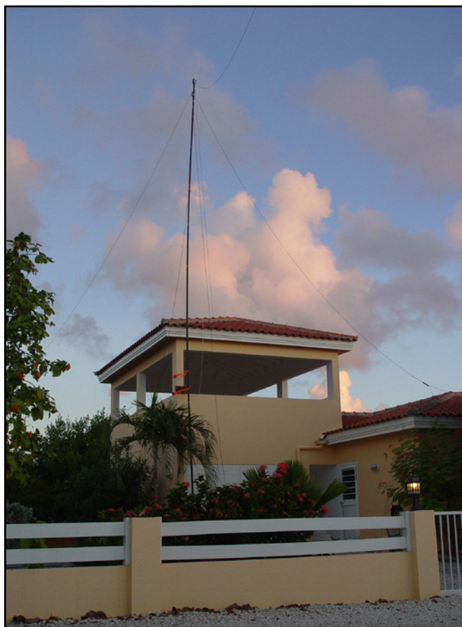
Newly installed 40- and 80-meter dipoles are draped from the 48-foot military mast. The support was originally to have been used to support two Yagis, but after trying in vain to find a way to guy the antennas, we ultimately scrapped the idea. After a week of using just a single station, this gave us two additional antennas and the ability to get our second operating position on the air.
